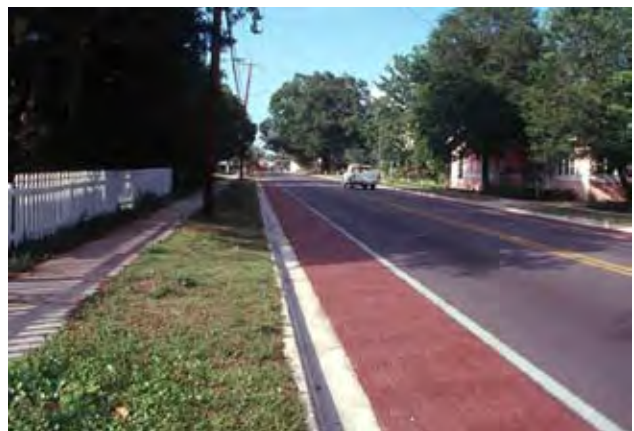
Example of a Complete Street along US 27 in High Springs, Florida Photos courtesy of Dan Burden. http://www.completestreets.org/
