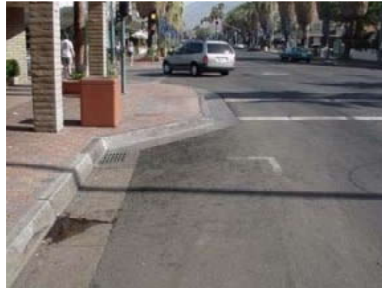
Figure 2. Curb extensions/bulb outs slow down traffic and provide safer crossings for pedestrians.
